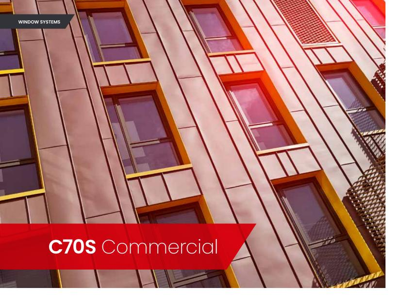
Beautifully engineered and brilliantly functional, the C70S delivers class-leading performance with U-values of 1.3 W/m2K, advanced water tightness and a range of features to simplify fabrication and installation.
